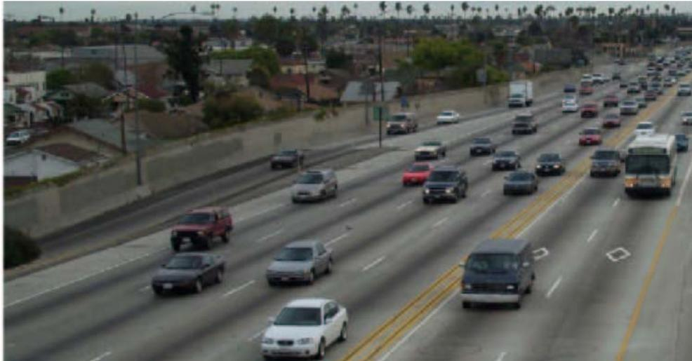
Figure 10. A concurrent flow HOV lane, marked by diamonds, in the offside lane (METRO, 2002)
