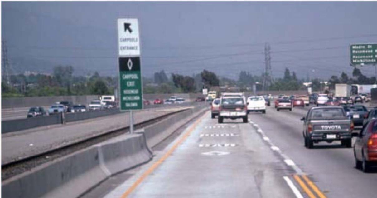
**Figure 1. A concurrent flow HOV lane in the offside lane (METRO, 2002a). This lane has no buffer.**
